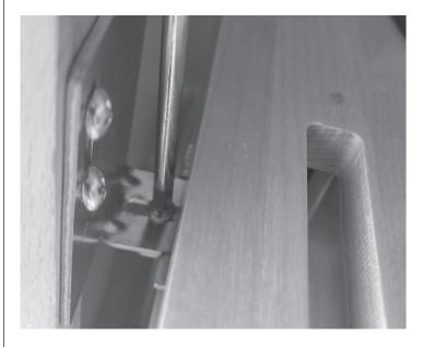
Pull and adjust the front L-Bracket into position onto the side of the face frame (or cabinet). Allowing for a 3/16'' setback. Firmly secure with two (2) #8 x 5/8'' Pan Head Wood Screws. Make sure the gap between the unit and the side of the face frame is equal from top to bottom. Adjust accordingly and then securely tighten the bracket set screw (shown with a screw driver). Operate the unit and make adjustments as necessary for the slides to operate smoothly.
