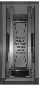
Place the slide base inside the cabinet, pulling the front cross member tight against the rear of the face frame. For frameless cabinets, set the front cross member back 3/4". For inset door applications, slide the base back from the above measurements plus the thickness of the door. Firmly secure with four (4) # 8 X 5/8" Pan Head Phillips Wood screws provided in the locations shown above. Replace the organizer onto the slide base. Proceed to the next step.
